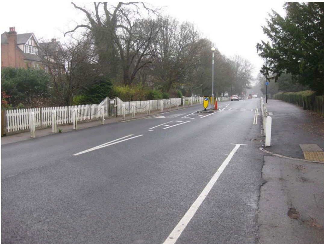
Pedestrian refuge protected by an existing short length of at any time waiting restrictions (double yellow lines) outside No.31
